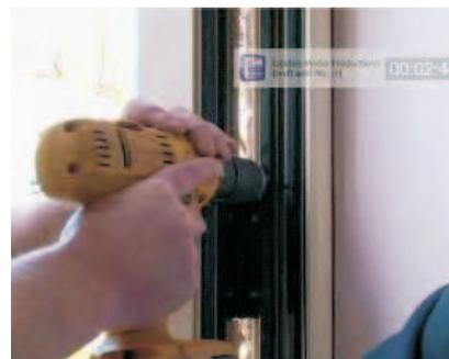
The fixings in the head and the cill should sit as flush as possible to enable the rollers to easily pass over the fixings but it is important that these are not over tightened as this will distort the aluminium track and prevent the door from operating correctly.
