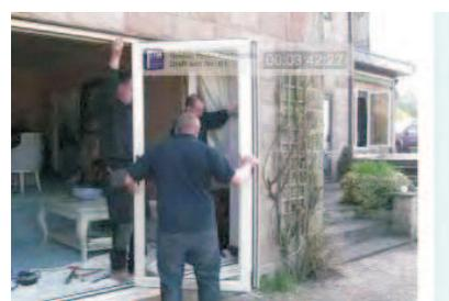
Carefully remove the beads from the first sash noting the position of each and position the glazing packers
