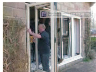
Fixing distances : corner fixings shall be a minimum of 150mm and a maximum of 250mm from the corner. Intermediate fixings shall be at centres no greater than 600mm.
